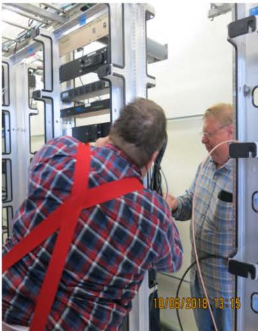
Keith and Joe (WA7JAW) wiring the repeater
